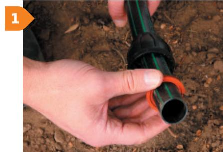
1 Cut the pipe square and place the nut and grip ring on to the pipe.
