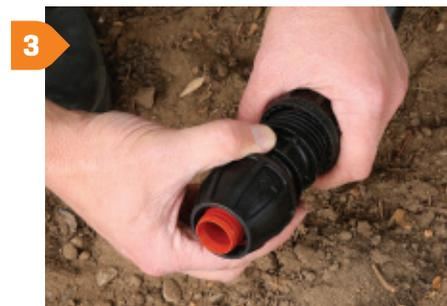
3 Position the insert in the body of the fitting, position the grip ring and nut and tighten by hand.
