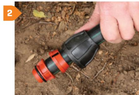
2 Tap the insert fully into the pipe.
